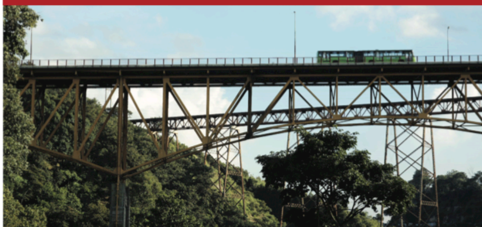
CoST Guatemala saved US$5 million through their intervention in the Belize Bridge project.
